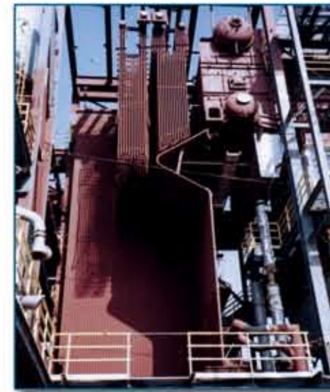
• 2-Drum Boiler being erected showing pendant Superheater •
