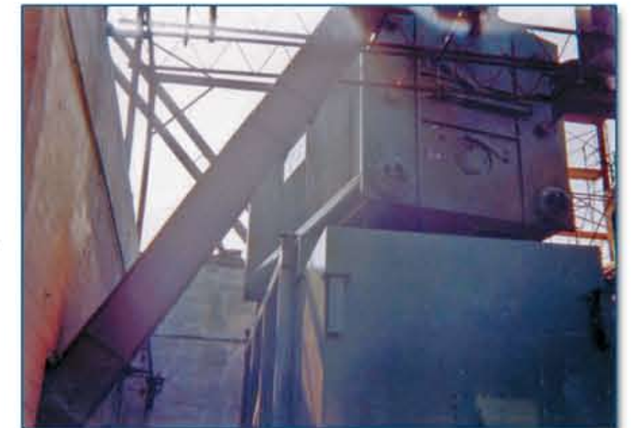
• A - Boiler being lifted into place •
